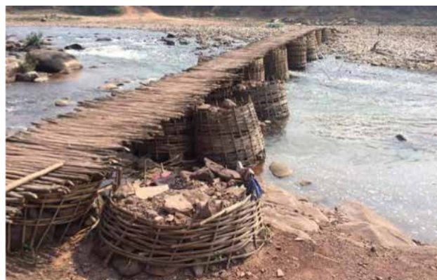
Figure 27 - Bridge in Samuoi District, UN Habitat, 2017
