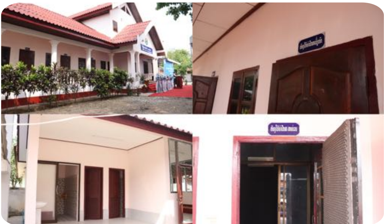
Protection shelter/One Stop Service Centre established in Attapeu
