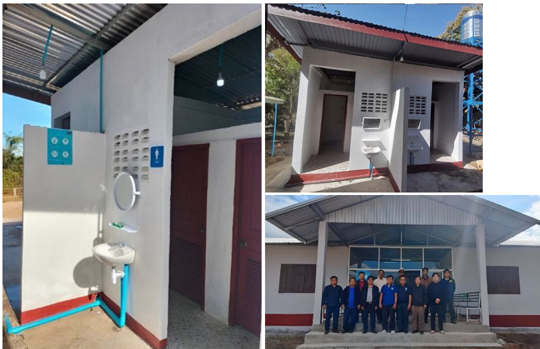
The Rehabilitated WASH Facilities
