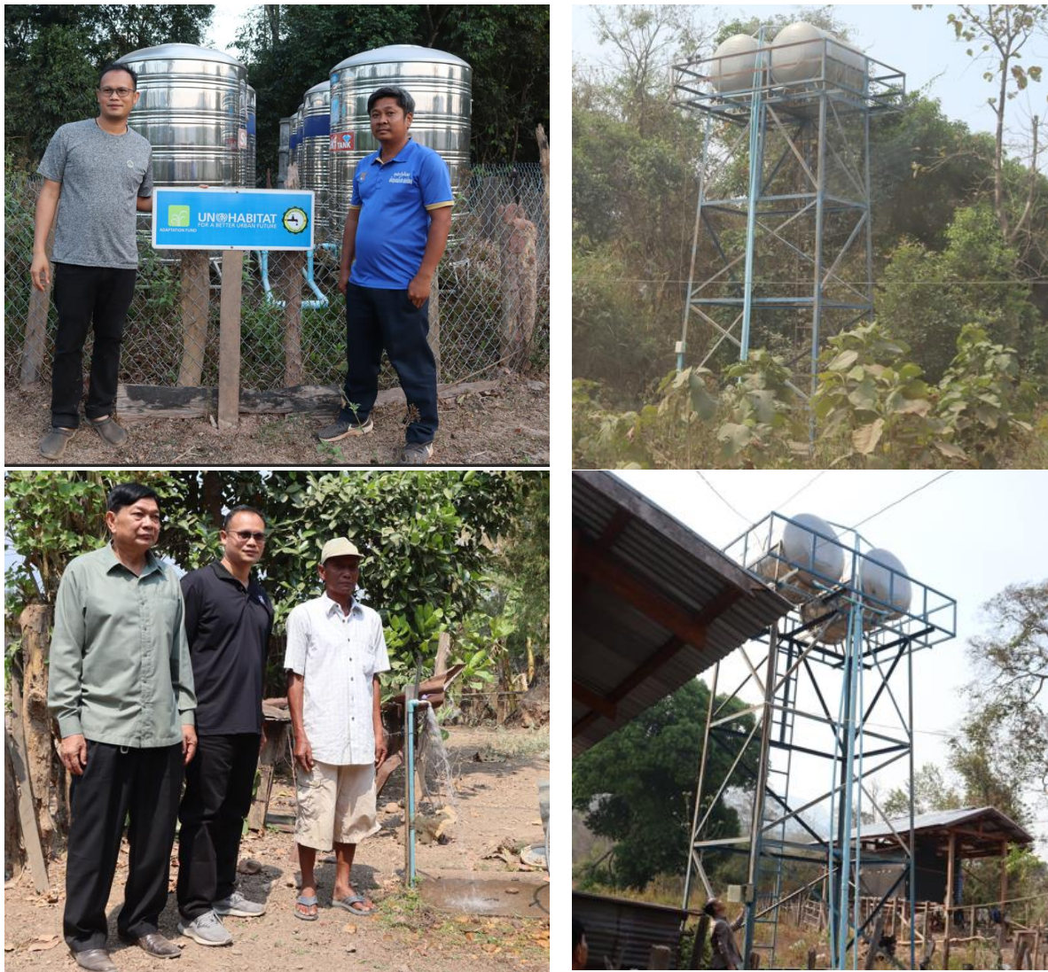
Figure 6: Water infrastructure built in Attapeu
