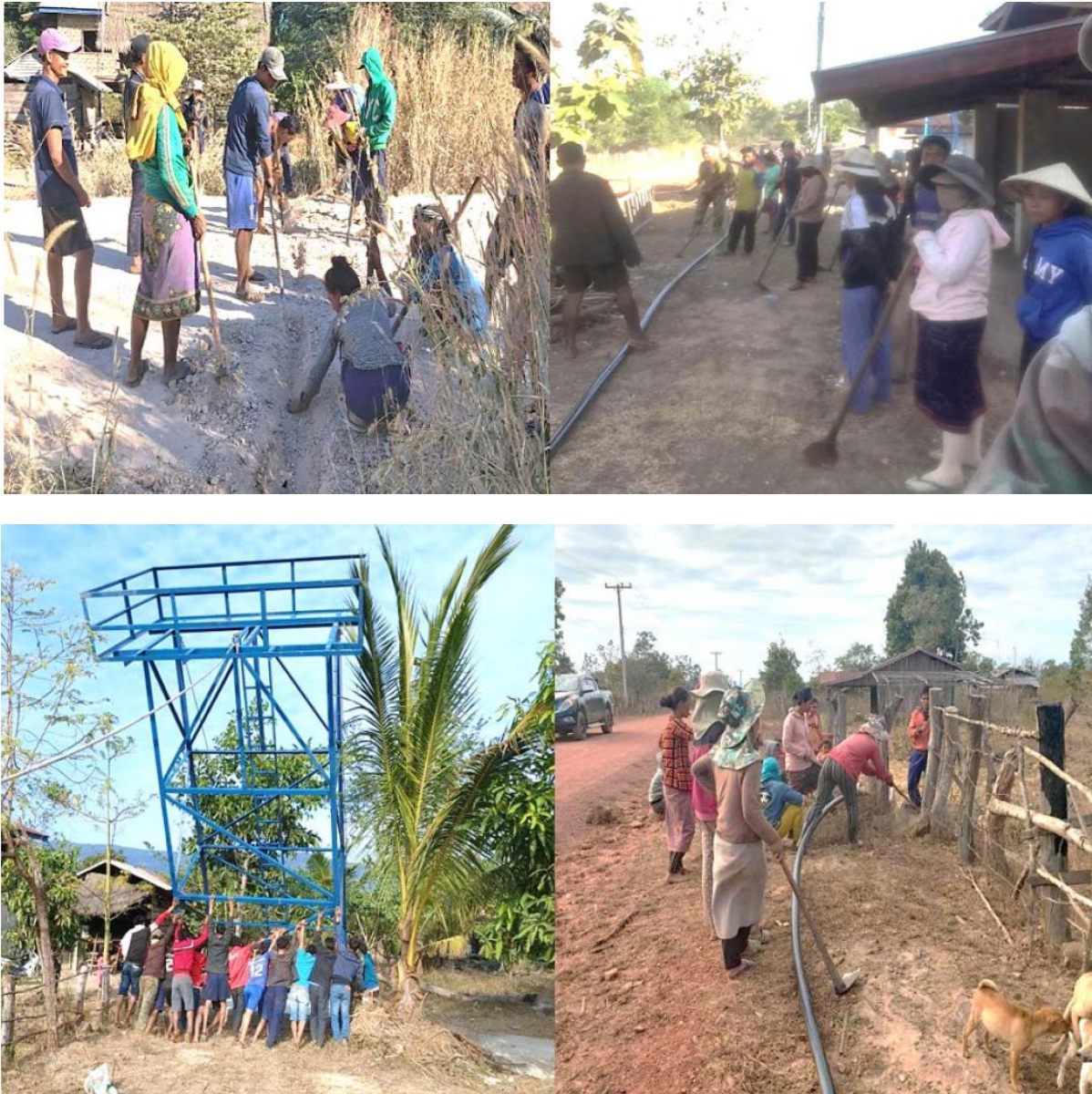
Figure 10: Community in-kind contributions by helping in digging and other excavation works
