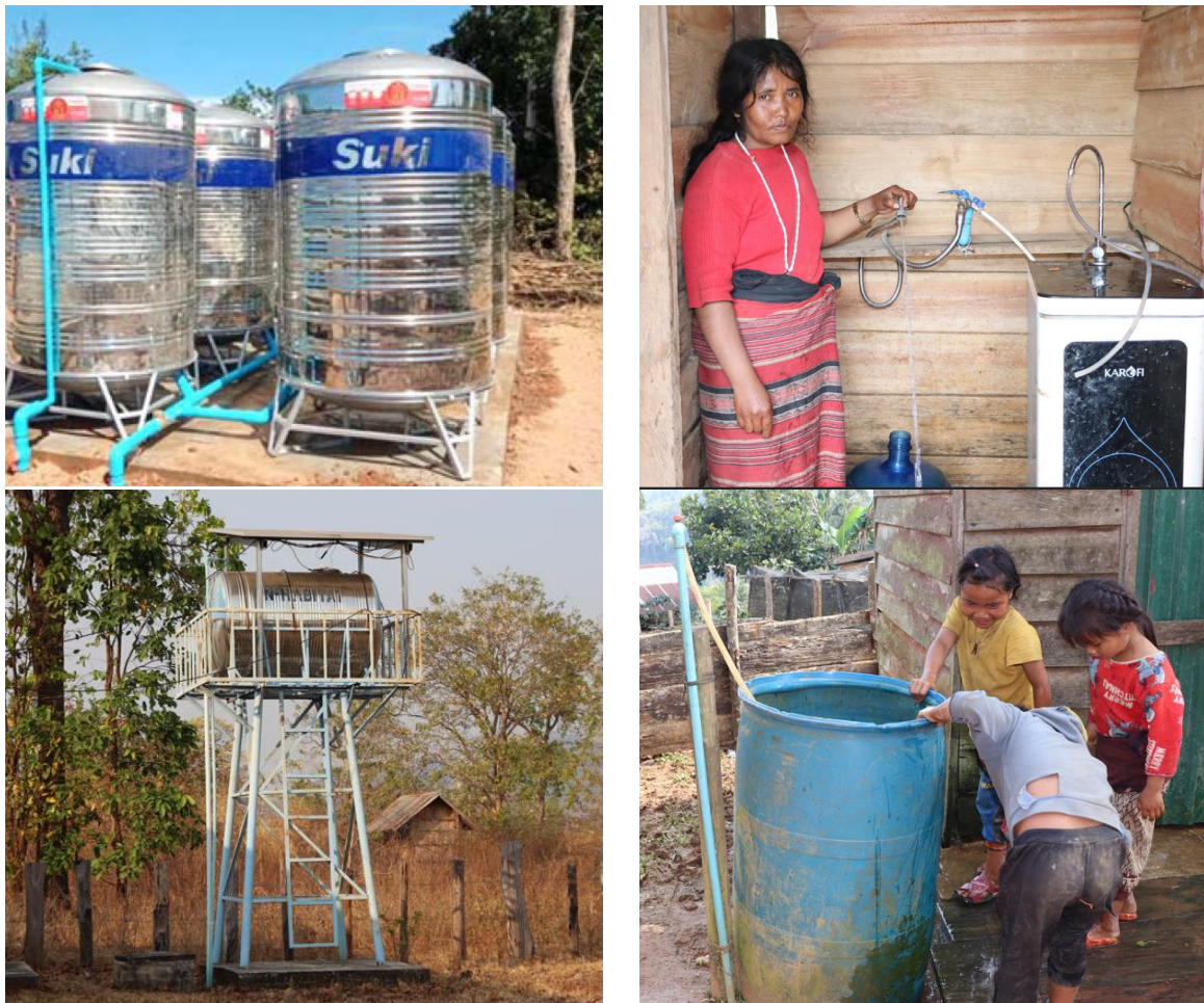
Figure 8: Water infrastructure built in Sekong
