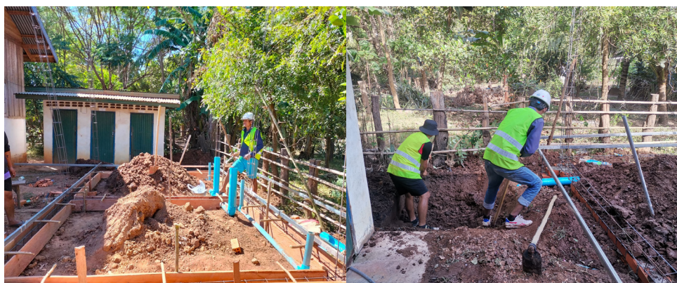
FIGURE 13. Construction Sites in Saravan Province, Safer Cities Project
